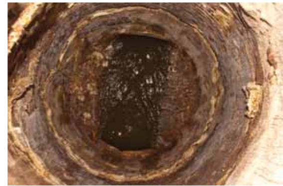
1. Manhole before being washed.
