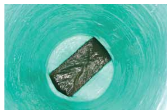
3. Manhole after being sprayed with Structure Guard.
