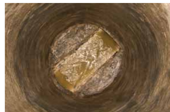
2. Manhole after being sprayed with Aluminaliner.
